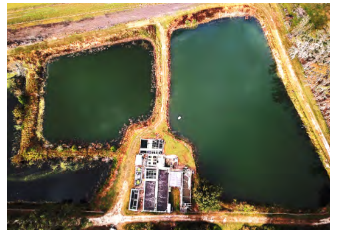
The retention ponds that receive processed water.
