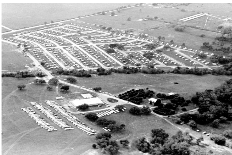
Aerial view of TR on Feb. 21, 1974.
