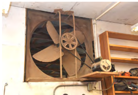
The need to keep the building properly ventilated is important. Sawdust from the use of the power saws, lathes, etc. filled the air with a fine powder that could be unhealthy.
