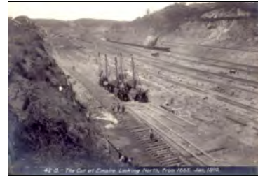
Digging out the main canal January 1910.
