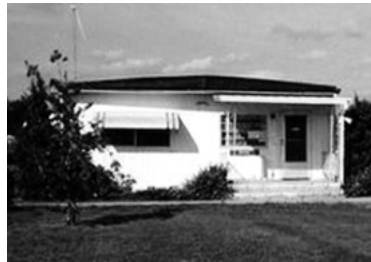
The first building that was purchased and put into place to be the TR Office. This was in use until June 2018.
