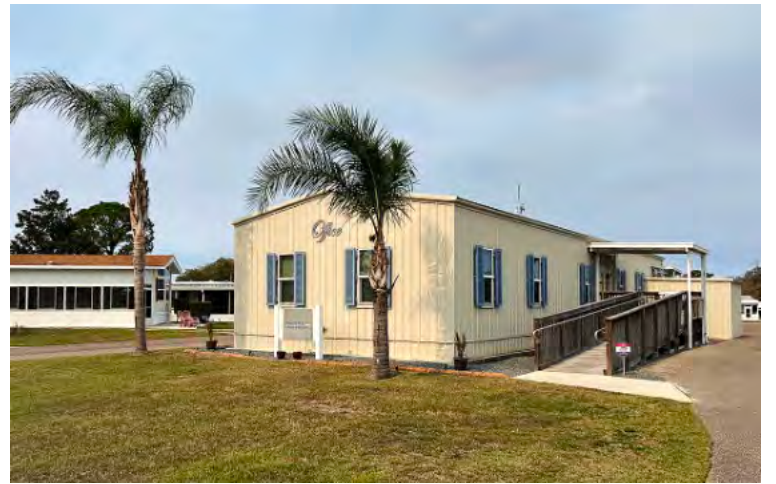
Our new Office complete with handicap ramp for easy access.
