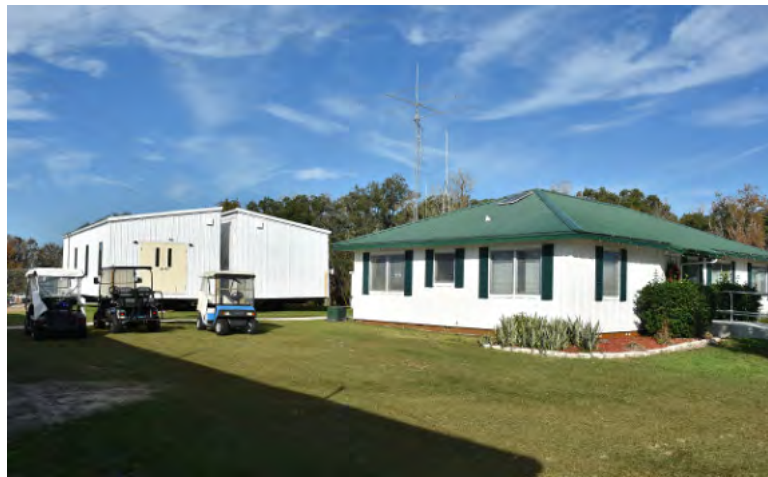
The building was delivered in two pieces and then joined together.
