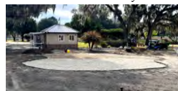
The design is taking shape as gravel and edging are added.
