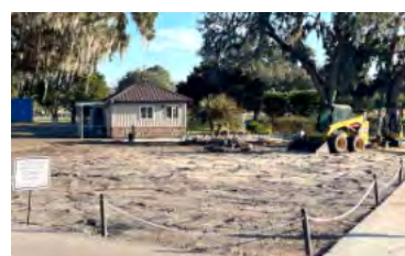
Front green removed in preparation for new design.
